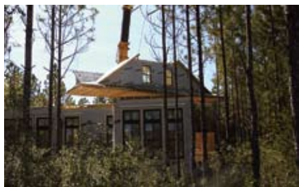
Modular building results in a healthy, energy-efficient home built in less time and with less waste than traditional construction methods.
